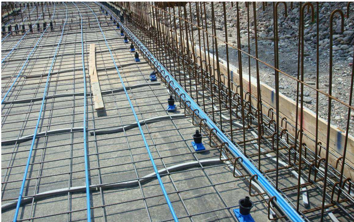
DD-1097A rectangular pocket former on 1E15 anchorage and DD 1095GK sealing gasket
